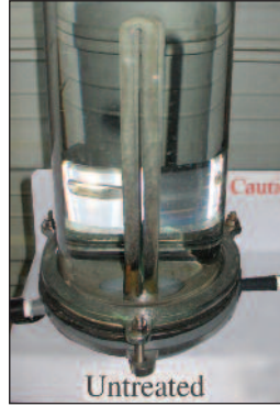
Scale Build-Up (In untreated water).
